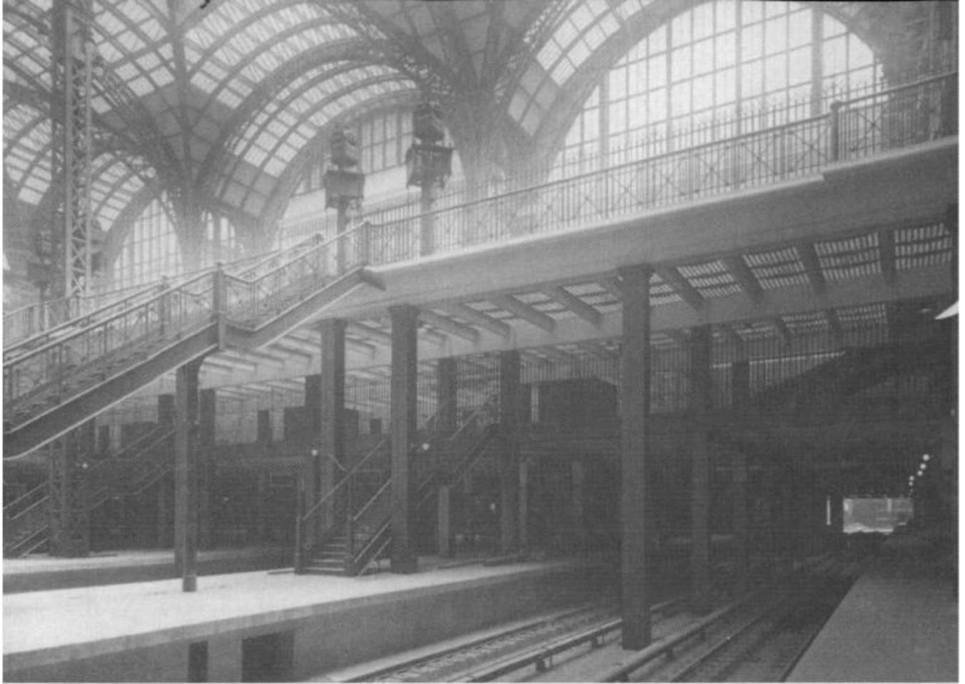
A 1910 trackside view in Penn Station just before service was inaugurated. (Library of Congress)
